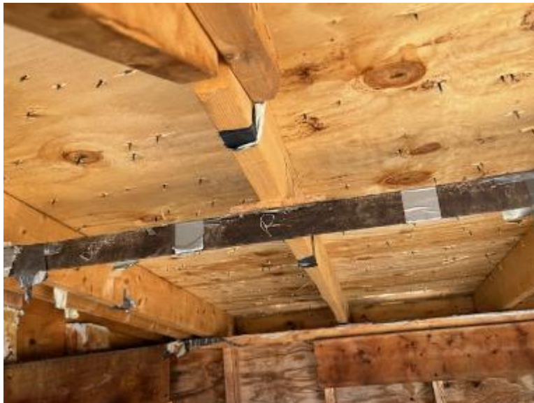
Photo No. 6 70 MPH Underside
