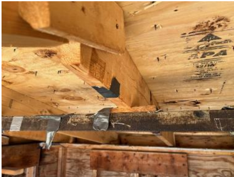
Photo No. 8 90 MPH Underside
