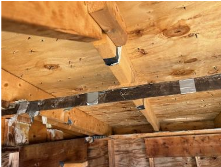
Photo No. 4 35 MPH Underside
