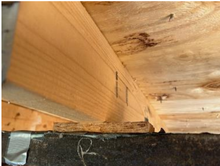
Photo No. 2 Underside Before Testing
