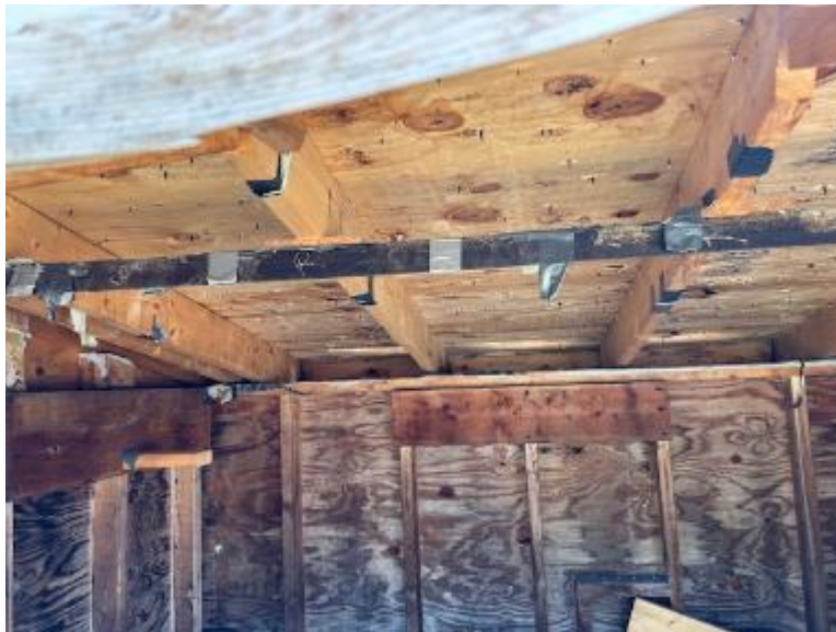
Photo No. 10 110 MPH Underside
