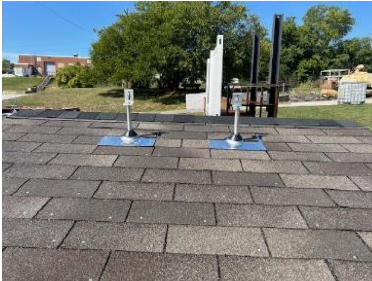
Photo No. 11 Post Test Top Side
